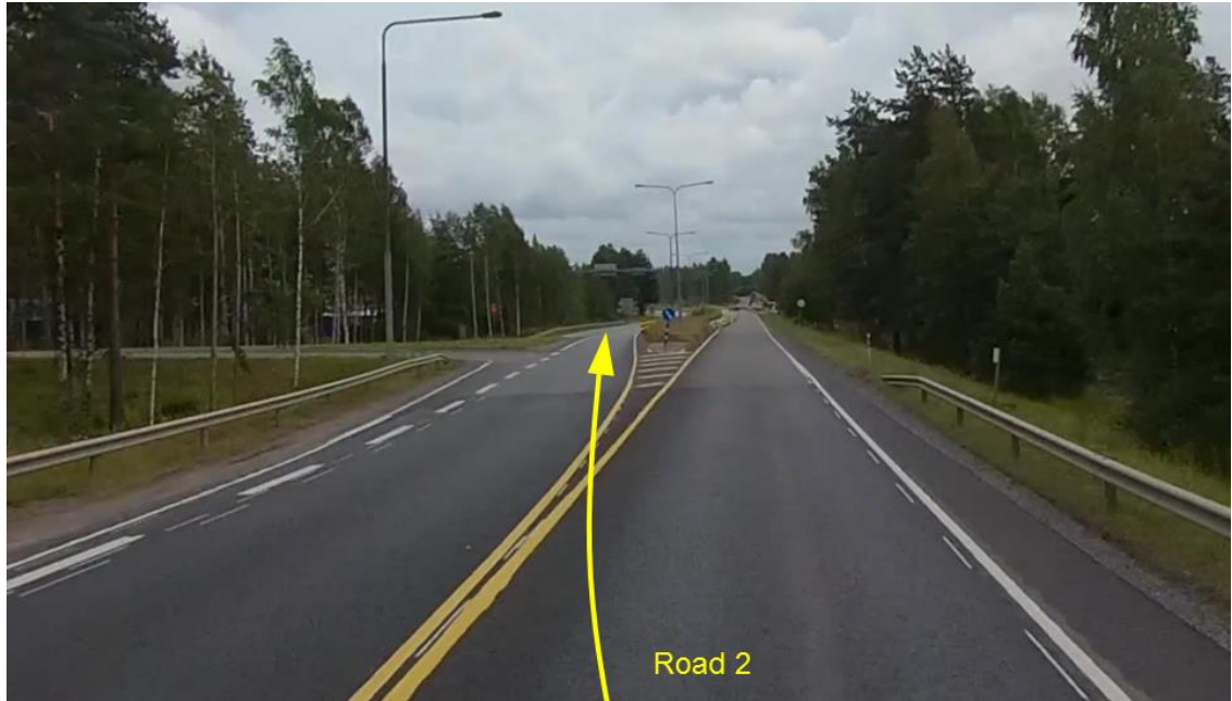
Figure 11: Transportations approach interchange road 2/road 8 facing the normal travel direction. 9
