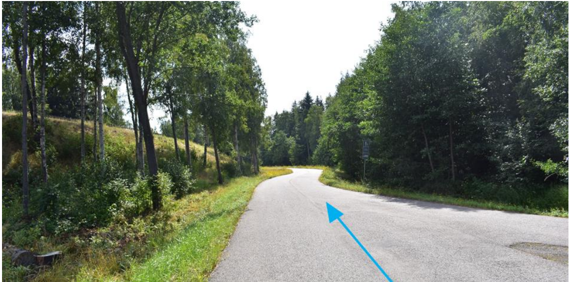
Figure 9: Route for transportations with height over 600 cm pass the bridge by cycleway which is meant to be used for abnormal transports. 7
