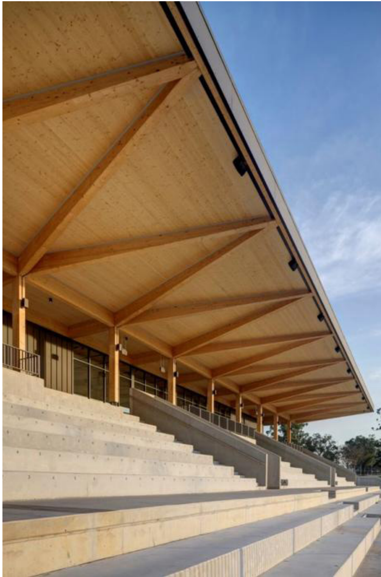
Eric Tweedale Stadium, Sydney, dwp / Northrop, www.northrop.com.au
